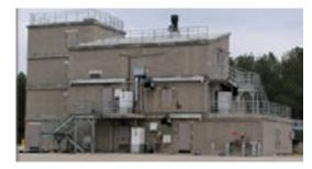
The Fire Research Building simulates a three-story residential structure with an attic, and a commercial structure with a basement. The building contains over 4,000 square feet of training space and is equipped with five computer controlled fire/smoke rooms with liquid propane gas fueled fire simulators, a Class A burn room, and a prop that simulates a couch fire with flashover capabilities. A four (4) story drill tower is attached to the burn area.
